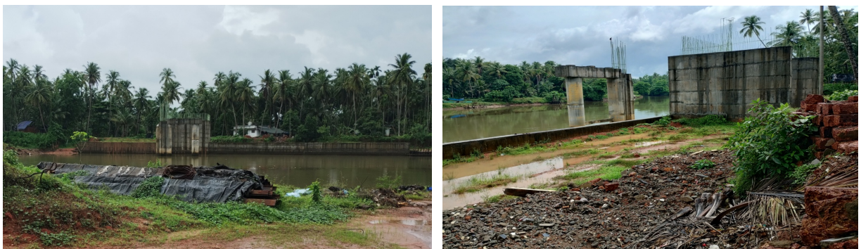
Regulator cum Bridge construction work is getting completed
