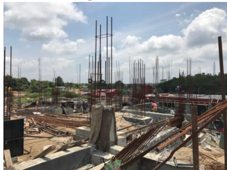
Transit Campus under construction
